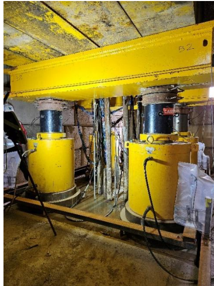
Plate 9: Hydraulic Jacks with Load Cells at Pile Head at LB-P1
