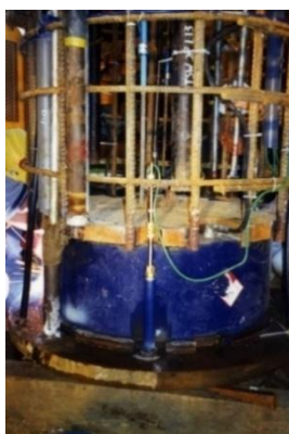
Plate 2: Osterberg Cell at Pile Base
