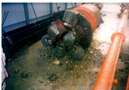
Plate 1: RCD for Construction of Rock Socket for the Test Piles
