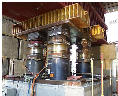
Plate 3: Hydraulic Jacks with Load Cells at Pile Head
