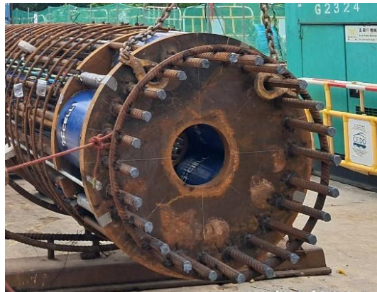
Plate 7: Underside of Bottom Steel Plate for LB-P1
