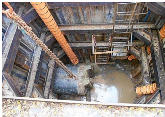
Plate 2: Shaft Excavation –Top View
