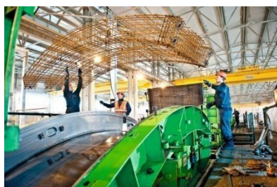
Plate 9: Steel reinforcement cage of tunnel segment
