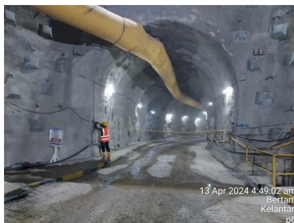
Figure 10: Reinforced Invert of the TCA
