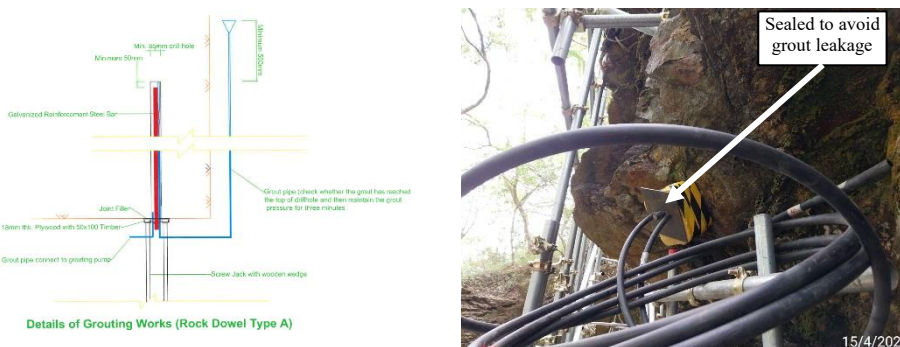
Figure 6: Details of grouting works (Left); Site photos of grouting of dowels (Right)
