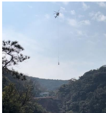
Figure 4: Helicopter Lift in Operation
