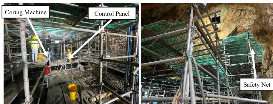
Figure 5: Coring Works - Scaffolding platform with safety net to prevent rockfall
