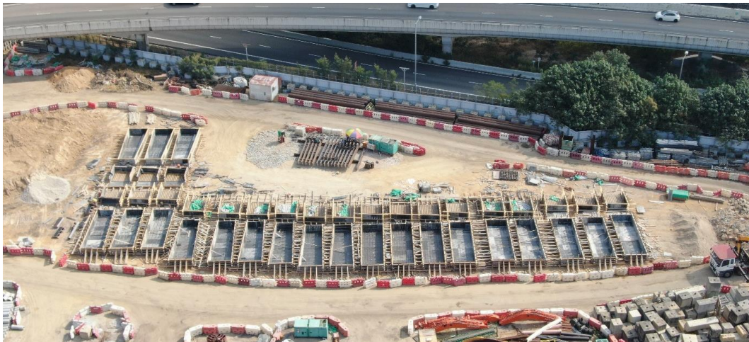
Figure 6: On-site casting yard
