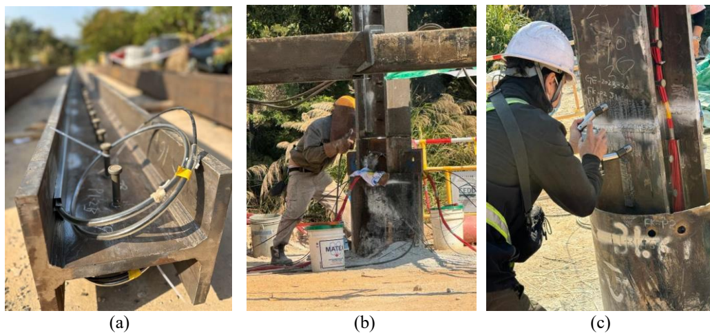
Figure 6.2: Construction details of trial piles with high strength S690 steel H-section: (a) Instrumentation with fibre optic sensors; (b) on-site welding; and (c) testing of weld.
